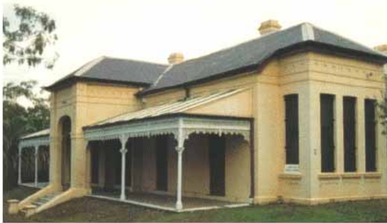
FIGURE 3: Linnwood demonstrates both local and statewide historic, social and aesthetic significance. Designed and built in 1891 by George McCredie, a prominent figure in both local and state politics, the residence is one of a very small group of residences in Holroyd of this architectural quality. In a statewide context the building is a good representative example of Victorian Italianate villa with much original fabric and detailing, at the local level it is a notably rare and fine example of such a building. The historic and aesthetic significance of the site is enhanced by the retention of some of its original landscaped grounds, which provide an attractive and historically appropriate setting for the main residence.
