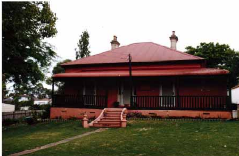
FIGURE 4: This house at No. 48 Albert Street Guildford demonstrates local aesthetic, social and historic significance. This property has historic and social significance as one of the earliest remaining large suburban residences constructed on the former “Sherwood” land, which was granted to William Sherwin in 1831. The property has aesthetic significance as one of the earliest remaining houses in Albert Street and as a fine and largely intact example of a Victorian Georgian style of building dating to the late nineteenth century. It also has aesthetic significance for the strong contribution the property makes to the character of Albert Street.
