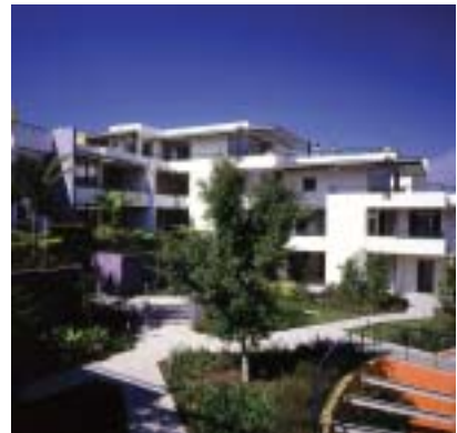
The site's topography has been used to create a series of smaller more intimate spaces using retaining walls and planter beds, which step down across the site.
