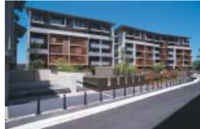
This facade has a strong balance of horizontal and vertical framing elements with sunscreens and balustrade infill components which gives it visual interest.
