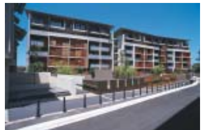
The detailing of the courtyard edge allows a visual connection between the street and the communal space, while clearly defining public and private realms.
