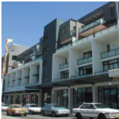
The facade of this building distinguishes the residential entry from the commercial shop fronts with a vertical element.
