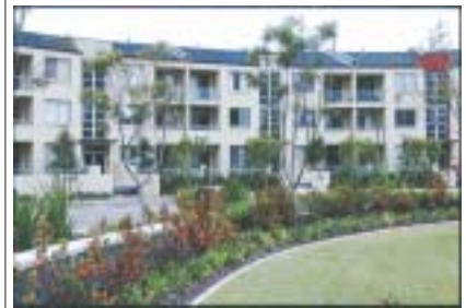
The use of multiple lift and stair cores promotes more number of entries along the street and thus helps in articulating a long building facade.
