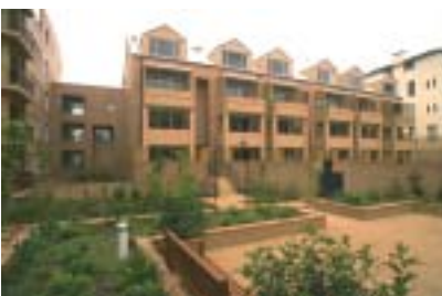
This facade is more traditional and uses a variety of repeated forms, and a restrained material palette.
