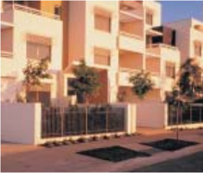
A picket and pillar fence defines the street boundary, clearly demarcating 'public' and 'private' space.
