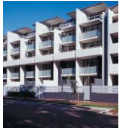
Lower level balconies have solid balustrades, limiting views from the street. Higher level balconies are set back beyond pedestrian sightlines and therefore glazed balconies are appropriate.
