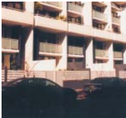
Multiple private entries along a street can activate the street and create visual interest.
