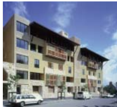
This facade has a distinct base, middle and top, and utilises materials which are sympathetic to the local context.
