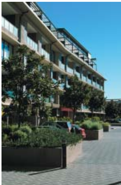
Where on-grade car parking is necessary, its impact can be reduced by quality paving and landscaping between smaller groups of car spaces.
