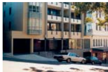
This small site on a steep terrain, has split the entry and exit driveways to maintain a consistent scale of facade openings.
