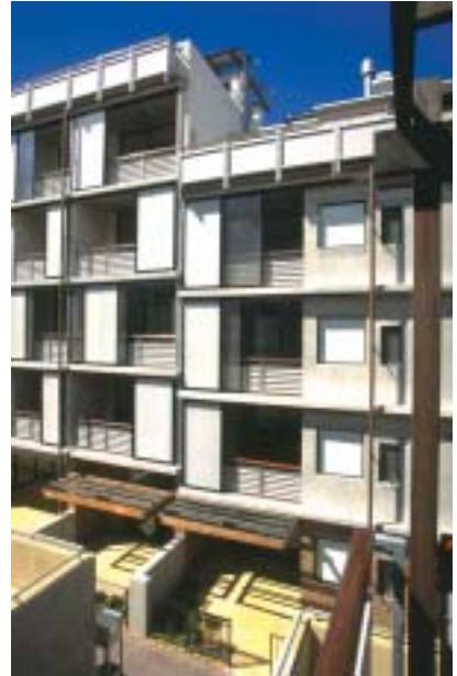
Building elements provide privacy between spaces, pergolas limit overlooking, solid walls and sliding screens limit horizontal views.
