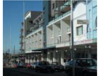
Variation in height of different floors adds to the articulation/visual quality of the building.
