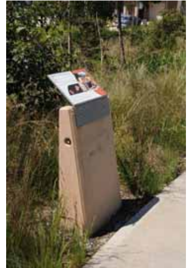
Figure 14 Trackside interpretive sign mounted on sturdy metal plate, bolted to concrete plinth. Photo: C Betteridge,
