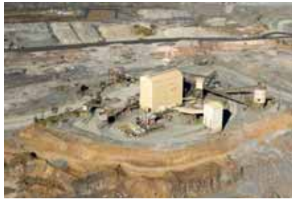
Extraction and crushing operations at Prospect Quarry, 2007.
