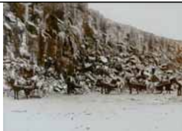
Quarrying at Prospect, 1900
