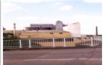
View north to Millmaster silos from Neil Street bridge.
