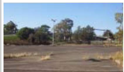
Part of block 4, which is currently being used as a car park, and is prone to flooding. The railway runs on the eastern side of block 4.
