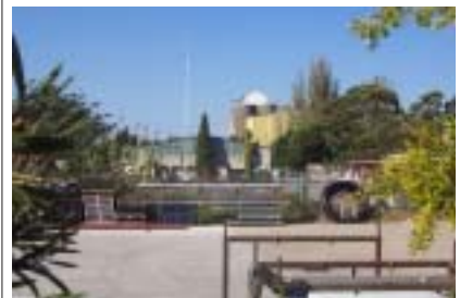
View from block 1 to Millmaster silos.
