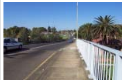
View east from Neil Street bridge.
